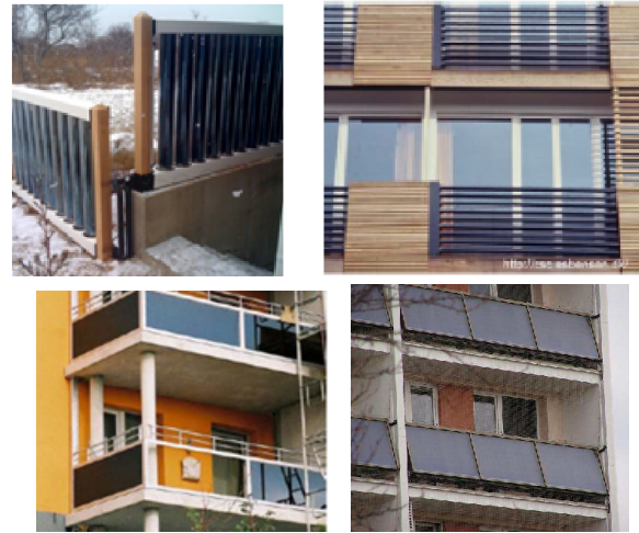
Fig.6. BISTS balustrade/railing feature
