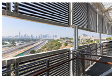
(e) Façade mounted evacuated tube collectors
